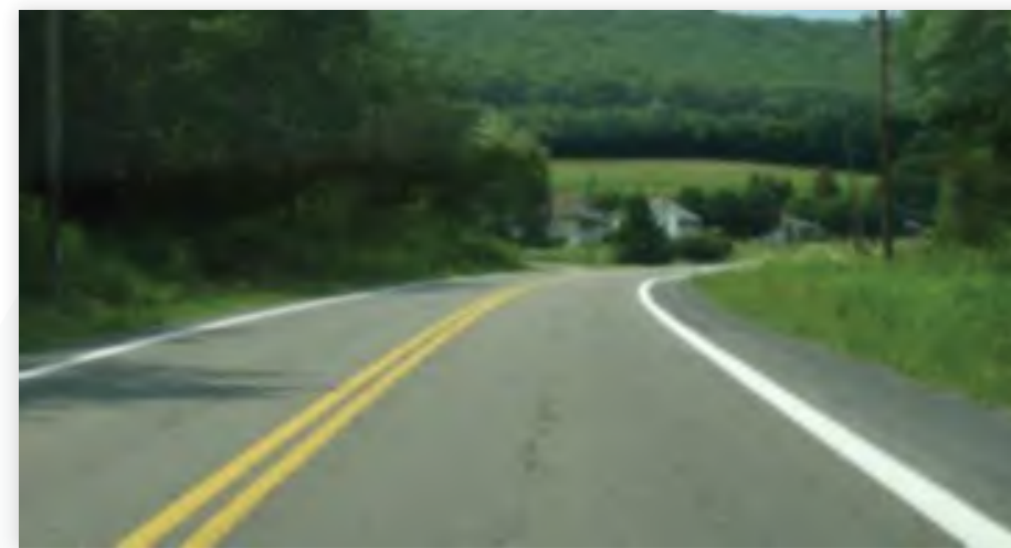
Wider Edgelines and Retroreflective Pavement Markings
